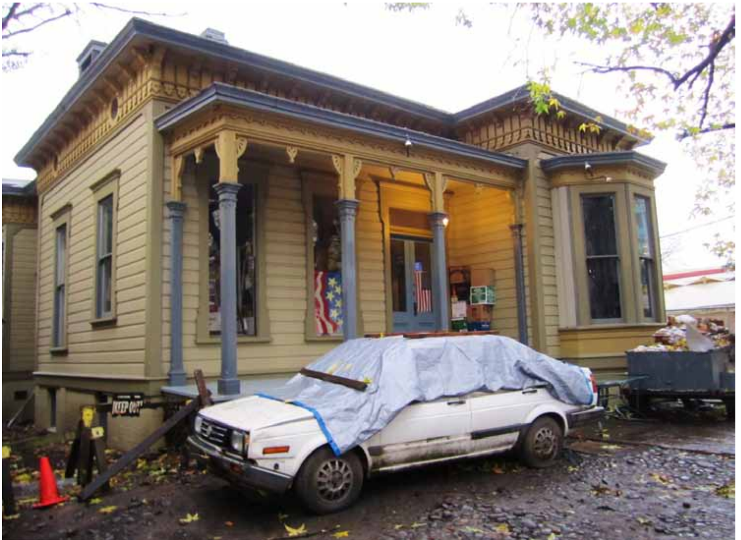
The Catlin Family's rented home at 120 (46) NW 21st Avenue. 1896-1901.
